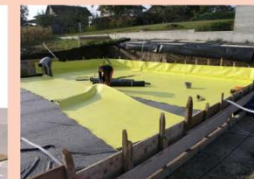
Detalj izgradnje vrlo niskoenergetske kuće drvene i betonske konstrukcije u Gorjupu / Detail of the construction of a timber-frame and concrete very low energy house in Gorjup, Croatia
