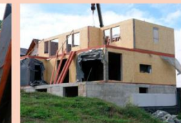
Vrlo niskoenergetska kuća MS (beton) gradnje / Prof. Ljubomir Miličević drvena i betonska konstrukcija u Gorjupu / Timber-frame and concrete very low energy house MS (beton) gradnje / Prof. Ljubomir Miličević structure in Gorjup, Croatia, under construction
