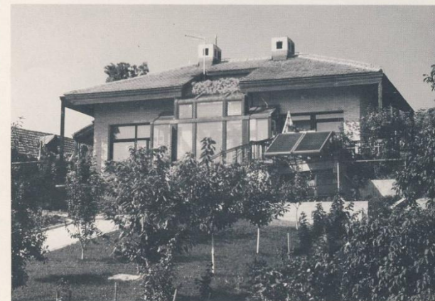
Fig. 1 House "P2" in Marija Bistrica 1985. South-east elevation and detail of the sunspace with massive stone wall
