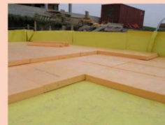
Detalj izgradnje vrlo niskoenergetske kuće drvene i betonske konstrukcije u Gorjupu / Detail of the construction of a timber-frame and concrete very low energy house in Gorjup, Croatia
