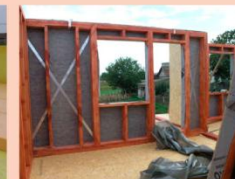
Detalj izgradnje energetske zgrade vrlo niskoenergetske kuće drvene i betonske konstrukcije u Gorjupu / Detail of the wooden wall installation of a timber-frame and concrete very low energy house in Gorjup, Croatia
